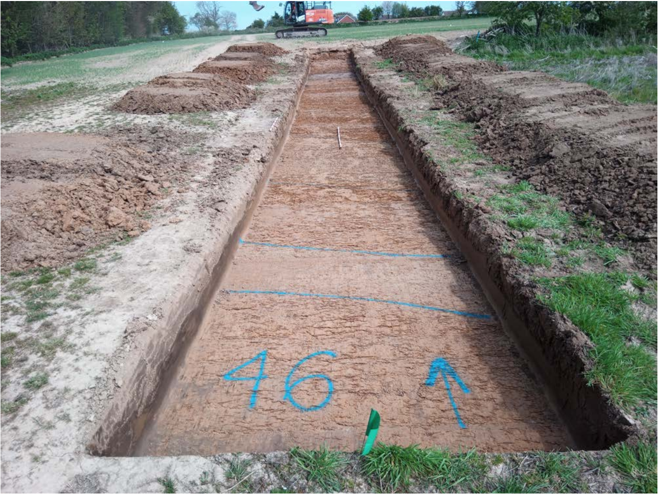
Plate 13: Looking north at trench 46; 2m scale.
