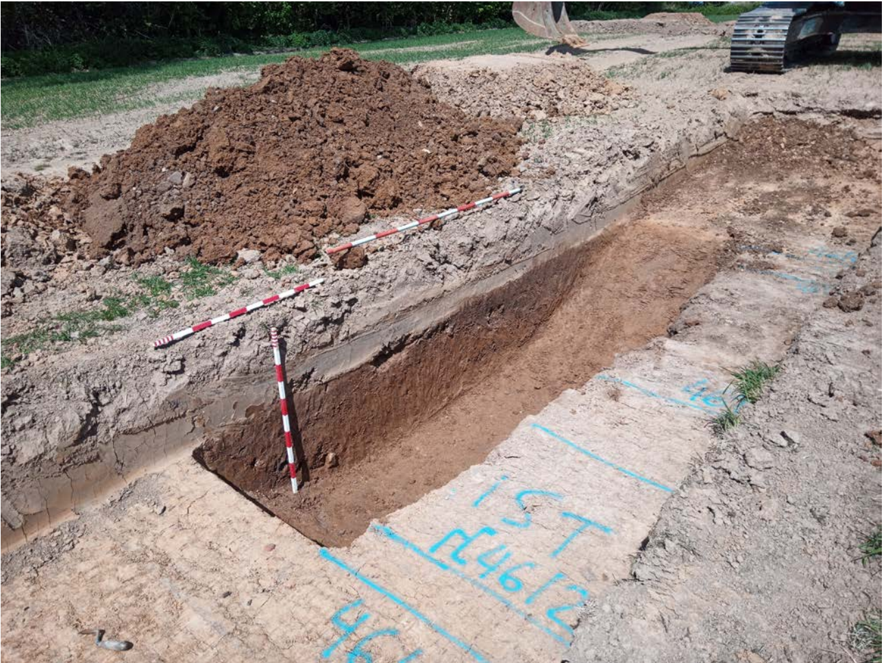
Plate 15: Looking north west at overcut section of ditch 4612 and modern ditch 4614.
